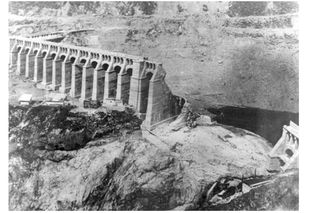
The Gleno dam a few days before the failure and the remains of the dam with the breach a few days after
