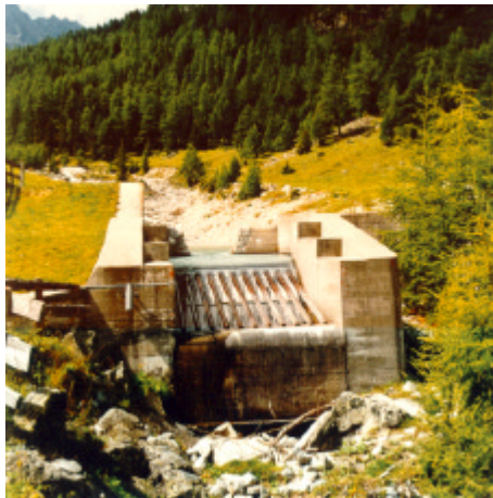
Figure 1: Tyrolean Weir of the water intake Verpeil, power plant Kaunertal
